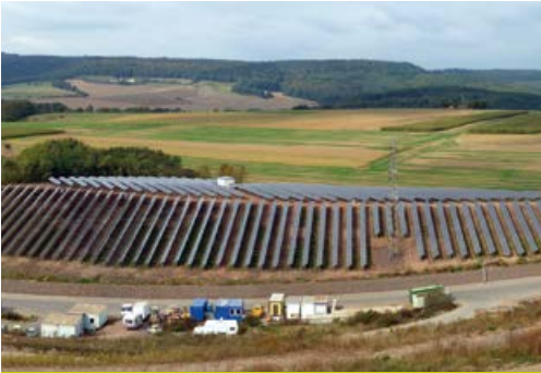
Large PV green field plant Sehlem Landfill
